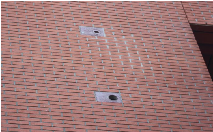
Image 3: Two nest boxes of different sizes on a building façade at GWL Terrain (Author, June 3, 2018).
