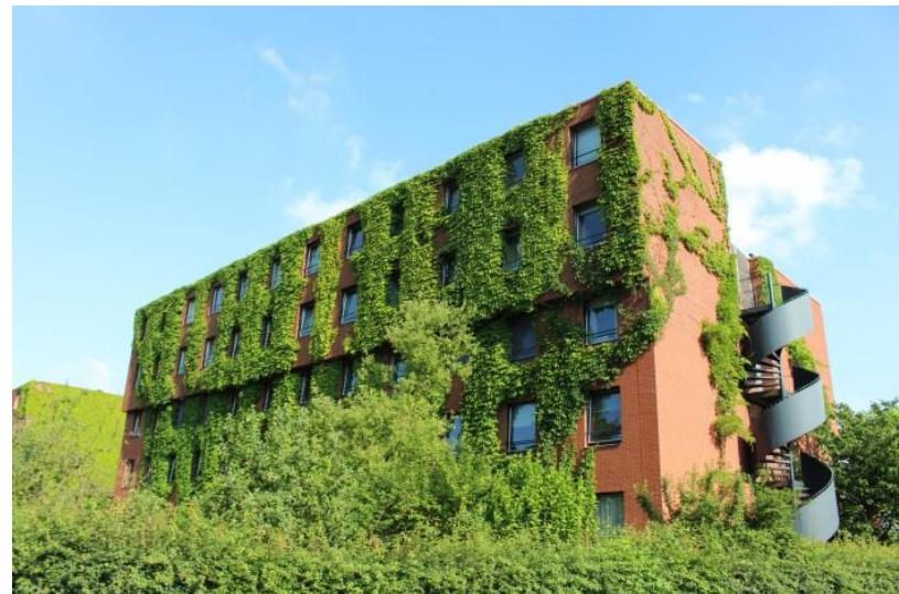
Image 6: Coarse vegetation on a building façade at GWL Terrain (Author, June 3, 2018).
